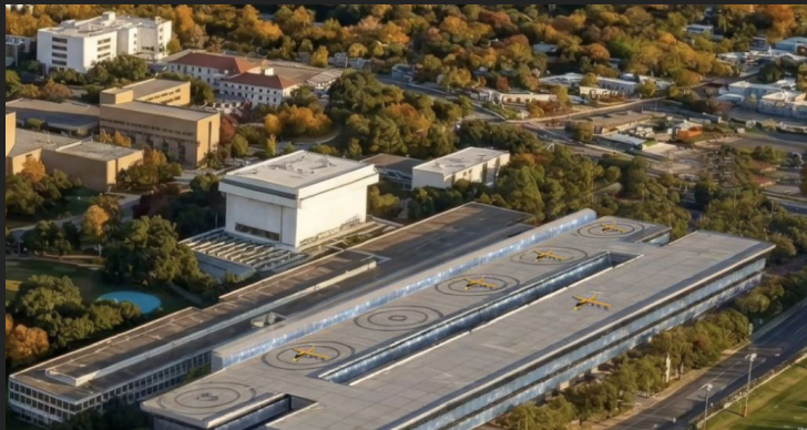
Rooftop Ultra Short Access Point in Urban Setting
